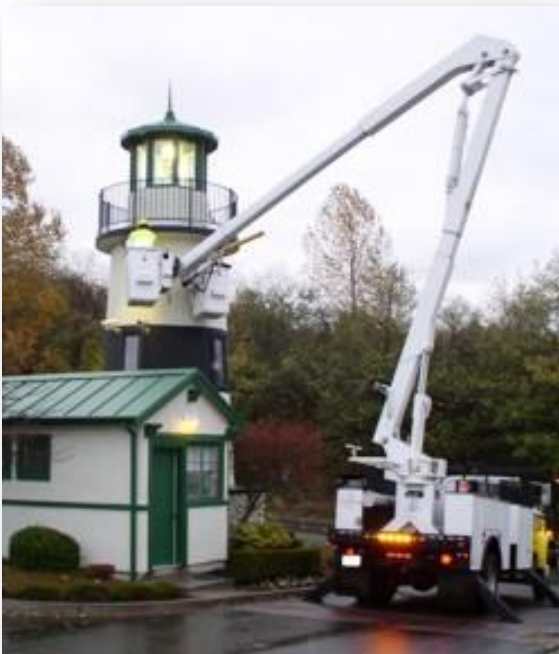
Equipment to do the Job
